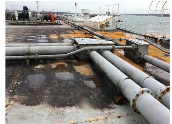
**Figures 71 and 72. Above, damage to the top deck above the garage. Below, exterior bulkhead on the port side of the garage while looking aft.**
