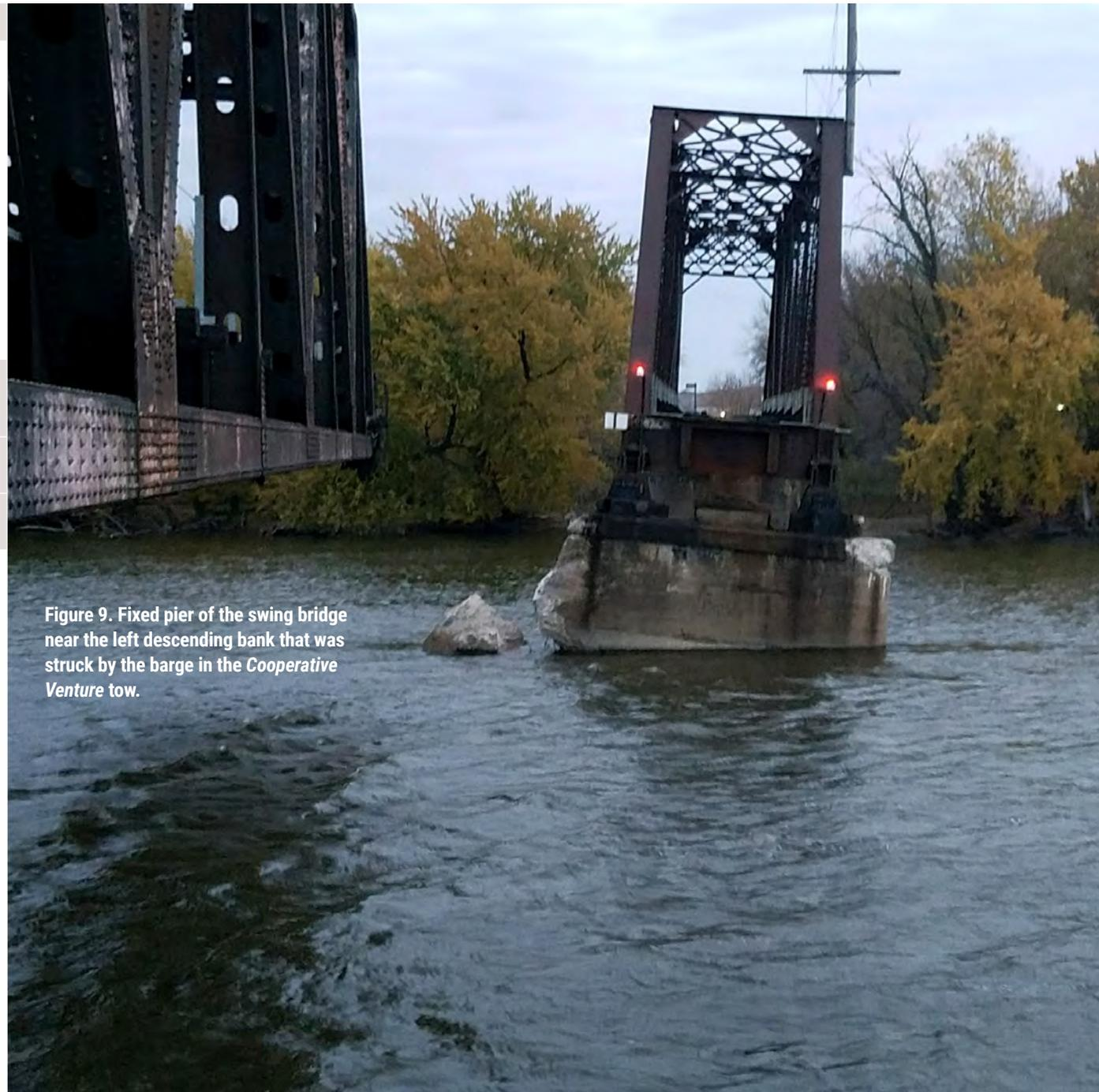
Figure 9. Fixed pier of the swing bridge near the left descending bank that was struck by the barge in the *Cooperative Venture* tow.
