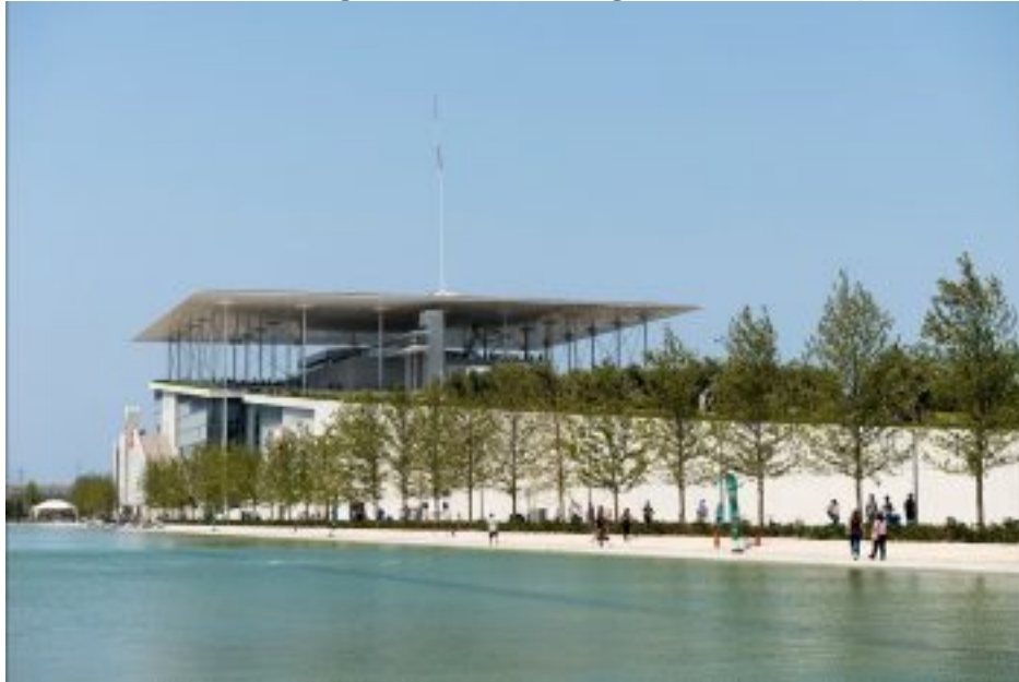
Stavros Niarchos Foundation Cultural Center (SNFCC). Photo Source:
