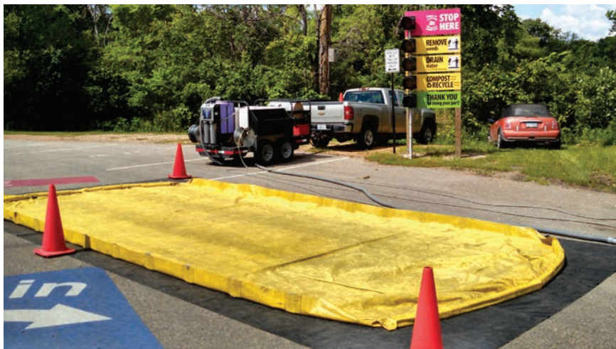
FIGURE 2- Example of a Portable Decontamination Station
